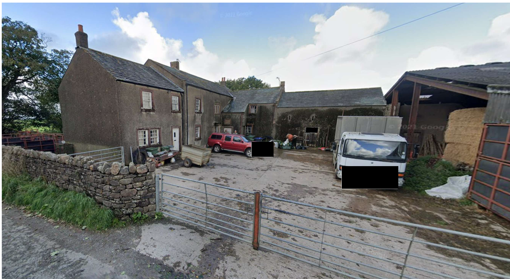
Figure 26: Crakeplace Hall 69 Grade II listed asset
