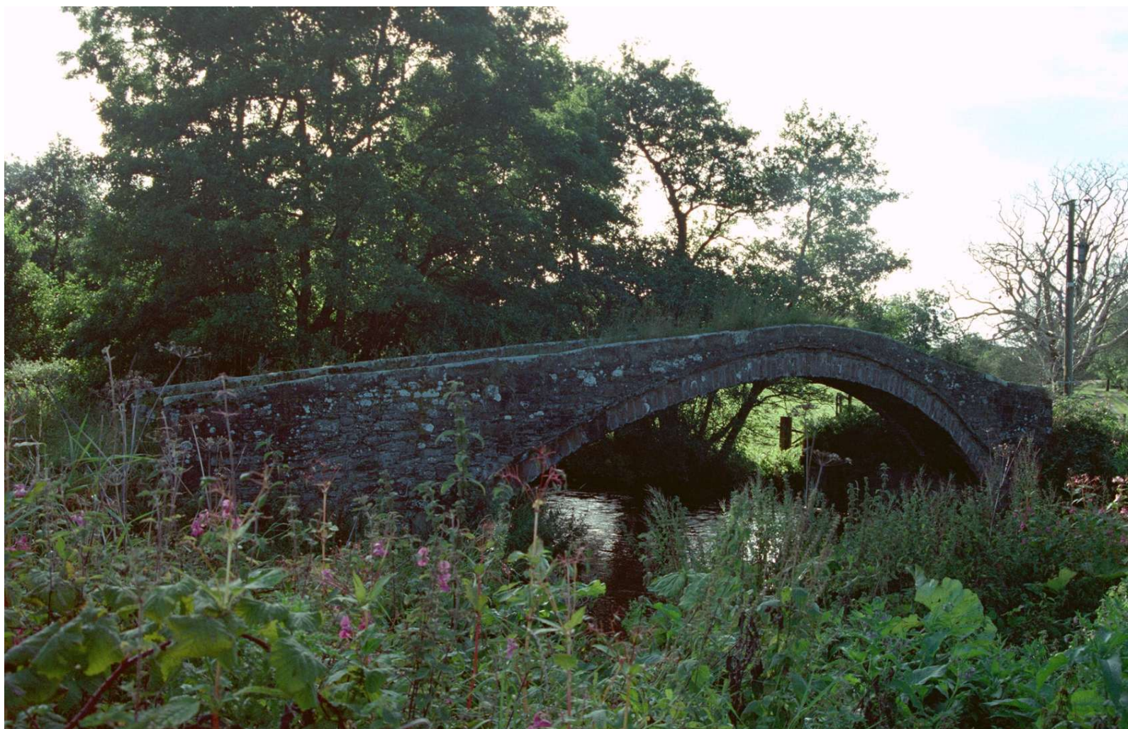
Figure 27: Calva Hall Bridge 70 grade II listed asset
